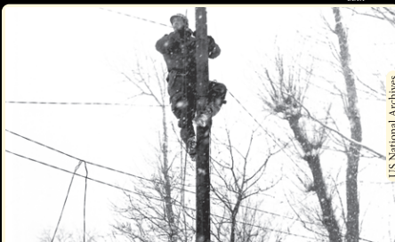
A lineman makes repairs to damaged communication lines.
